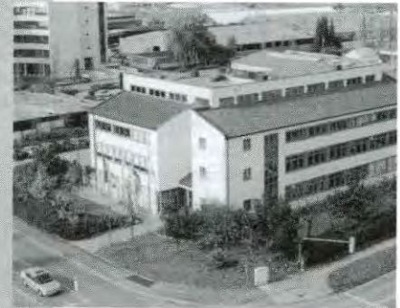
SV Headquarters building, Augsburg.
